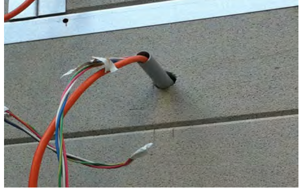
Hole penetration to allow cable and pipe access.
