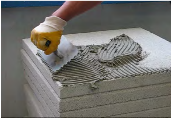
Apply adhesive on to the tile, with the notched edge of the trowel, preferably in one direction.
