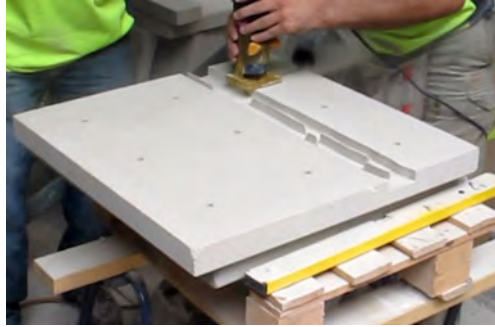
Hole penetration to allow cable and pipe access.
