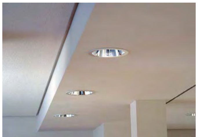
Reapor tiles rendered for an even jointless look.
