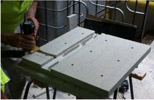
Reapor routed to allow cable access
