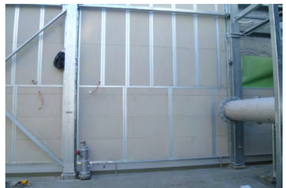
Reapor tiles installed using J-Channels
