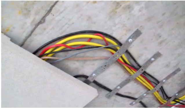
Reapor routed to allow cable access
